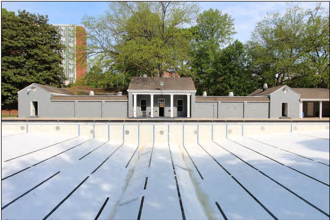
Figure 3.12 Pool House and pool (foreground), facing northwest.
