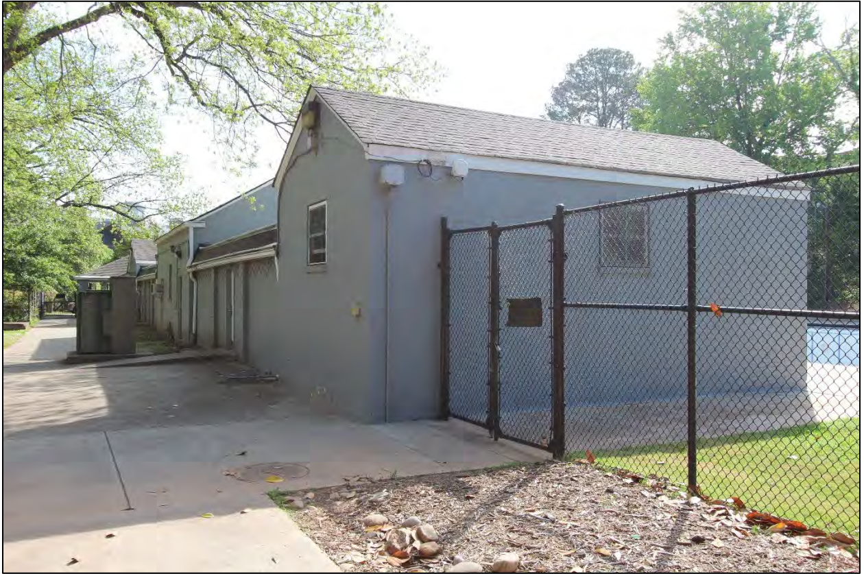
Figure 3.8 Pool House, southwest elevation, facing northeast.
