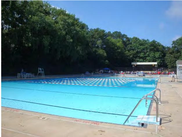
Image 3: Swimming Pool Structure
