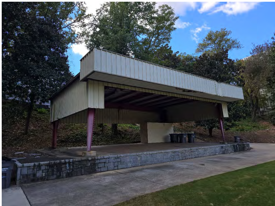
10. No hazardous materials identified with the existing concert stage
