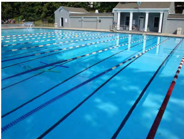
Image 11: Pool Main Drains
