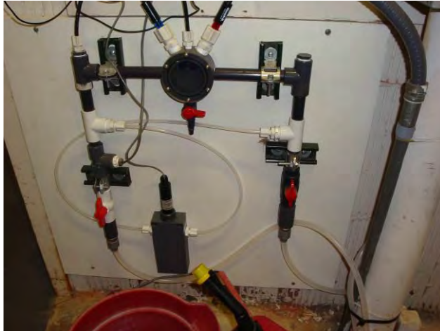
Image 86: Sample Stream & Probe Assembly
