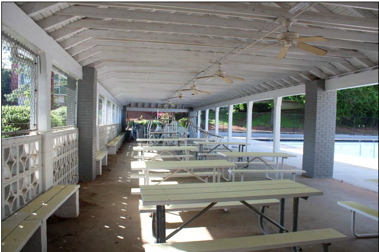
Figure 3.21 Pool House, pavilion area, facing southeast.
