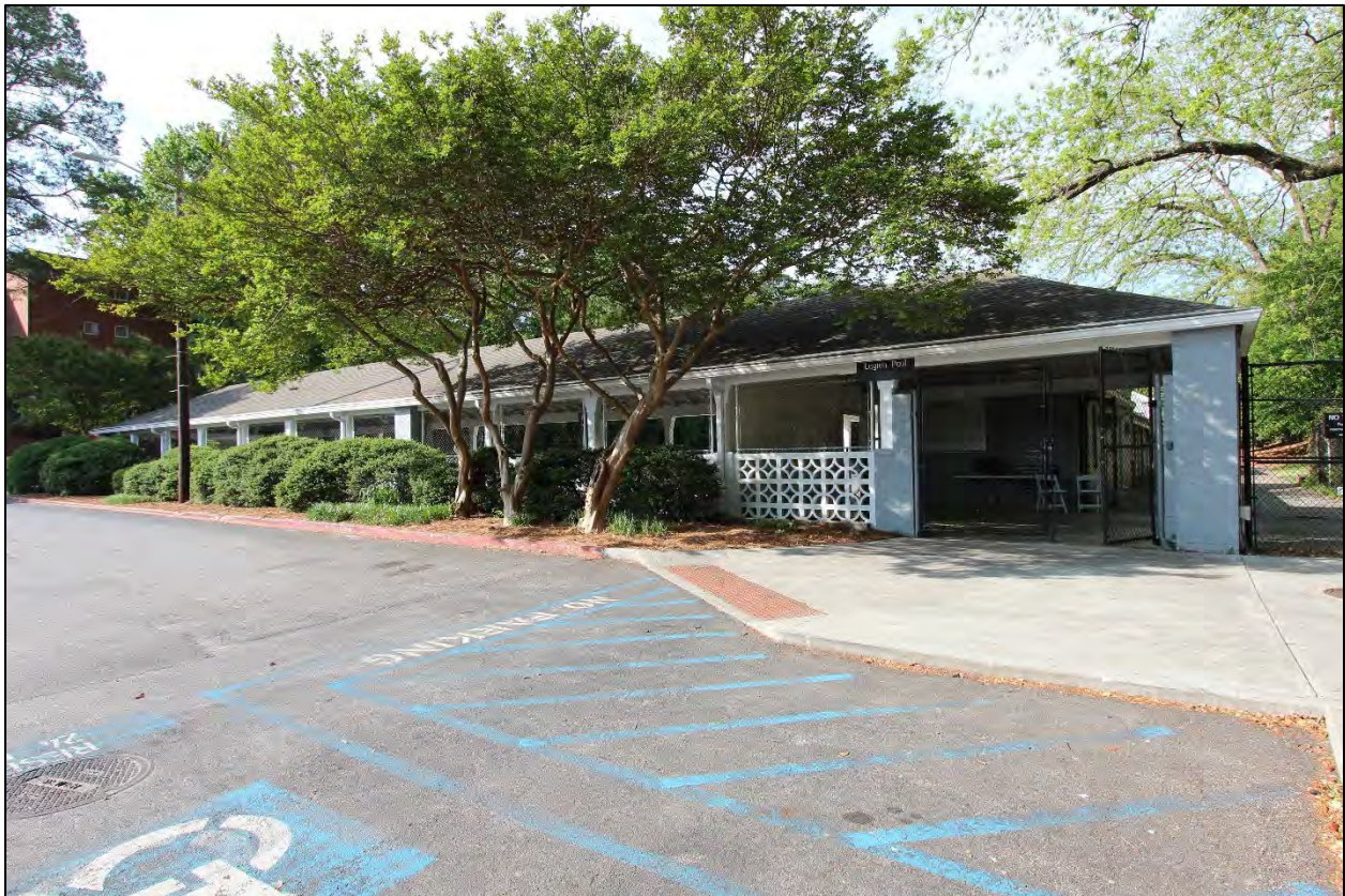
Figure 3.1 Pool House, near entry, facing south.
