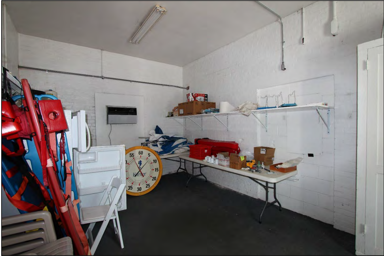
Figure 3.28 Pool House, central block, storage area.
