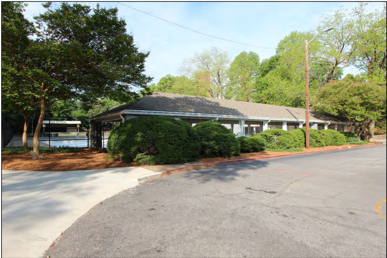
Figure 3.2 Pool House, facing southwest.
