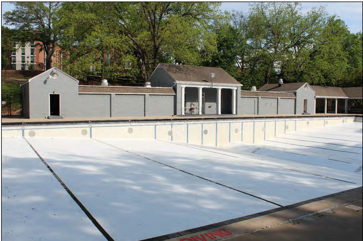
Figure 3.13 Pool House and pool (foreground), facing northwest.
