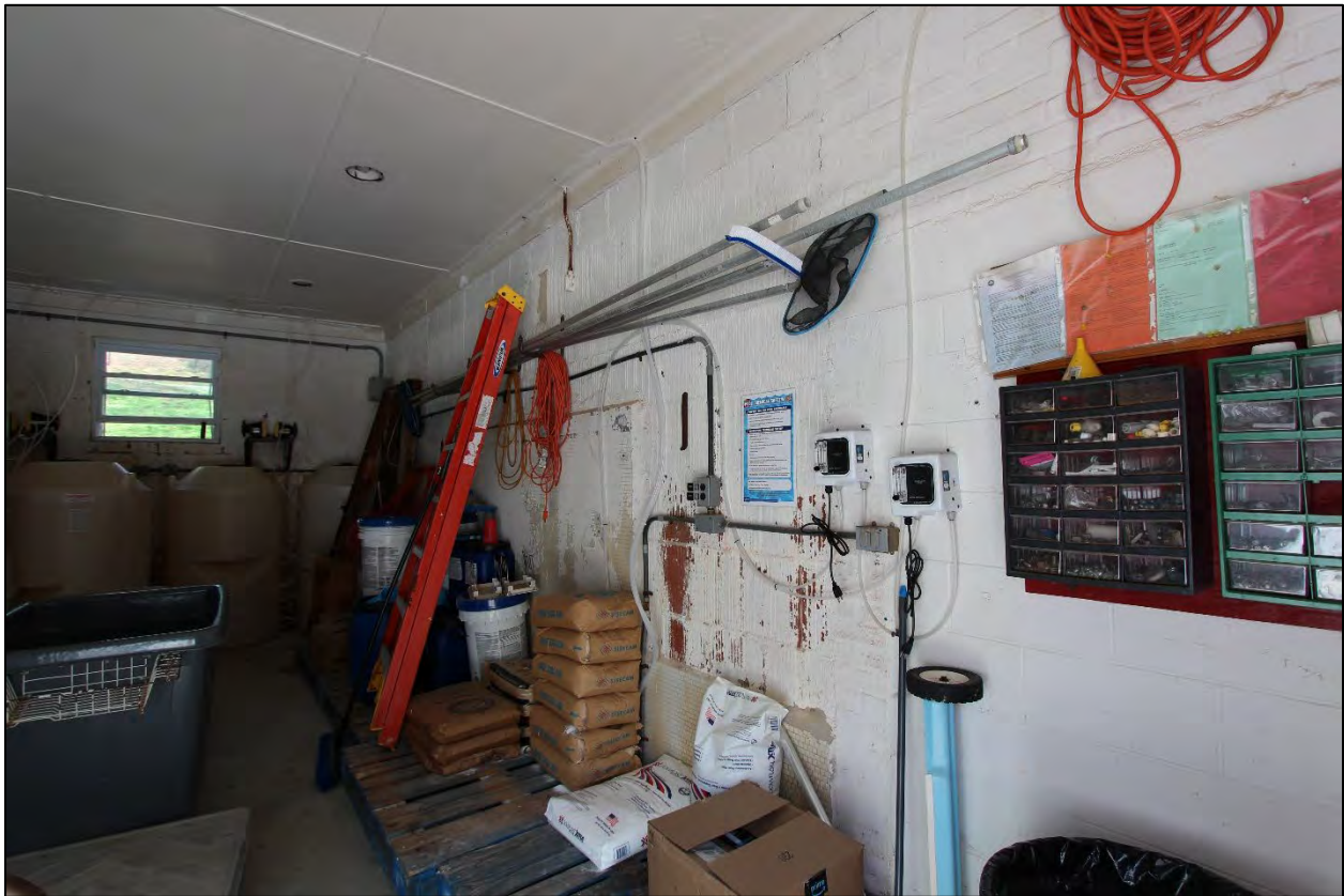
Figure 3.24 Pool House, southernmost wing, showing interior.
