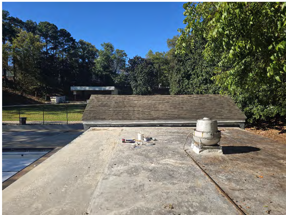
4. ACM BUR under TPO on Pool House (Flat Roof 2)
