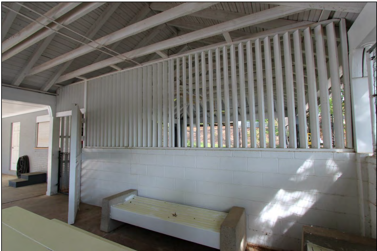
Figure 3.23 Pool House, pavilion area, showing louvered wall, facing northwest.
