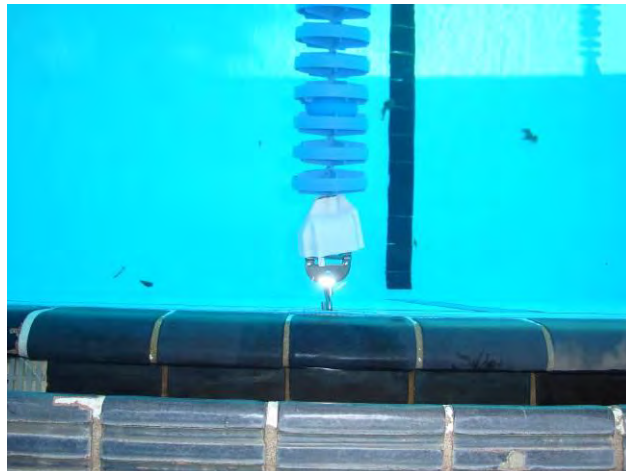
Image 23: Lane Marking & Rope Anchor
