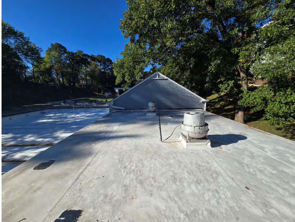
3. ACM asphalt built-up (BUR) roof under TPO on Pool House (Flat Roof 1)
