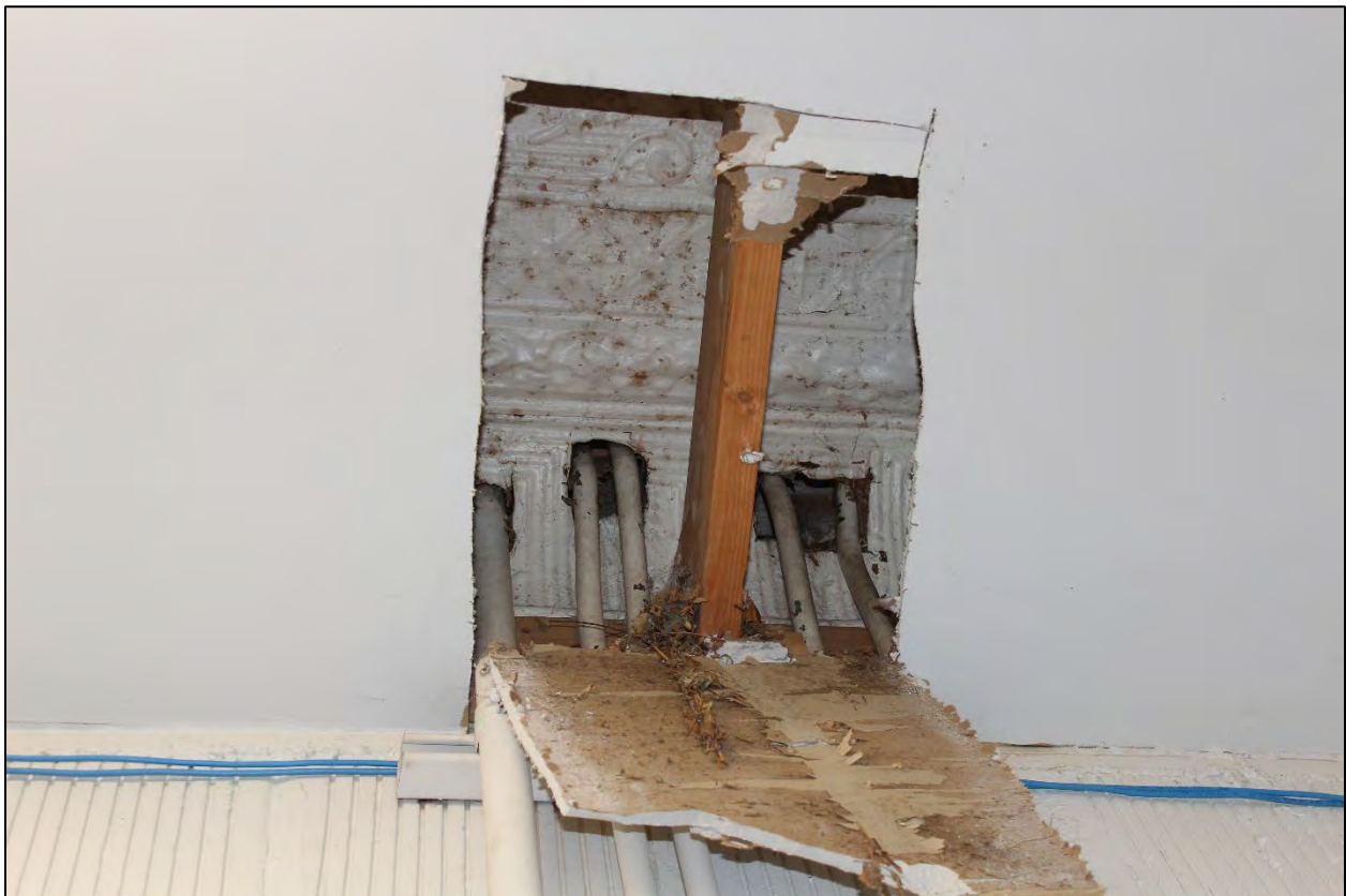
Figure 3.29 Pool House, central block, rear storage area, showing remnants of pressed metal ceiling.
