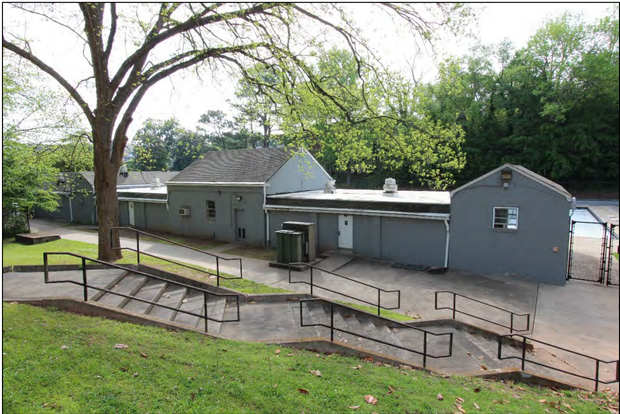
Figure 3.6 Pool House, rear elevation, facing east.
