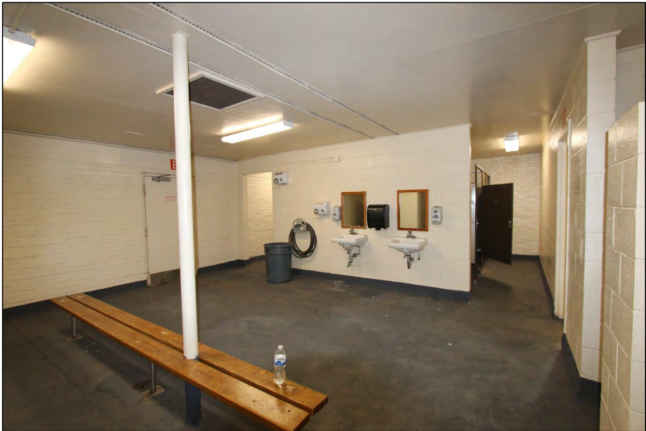
Figure 3.26 Pool House, men's changing area.
