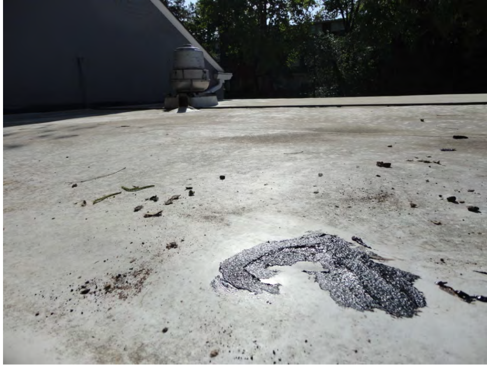
3. ACM built-up asphalt roof atop enclosed concessions/bathhouse structure.
