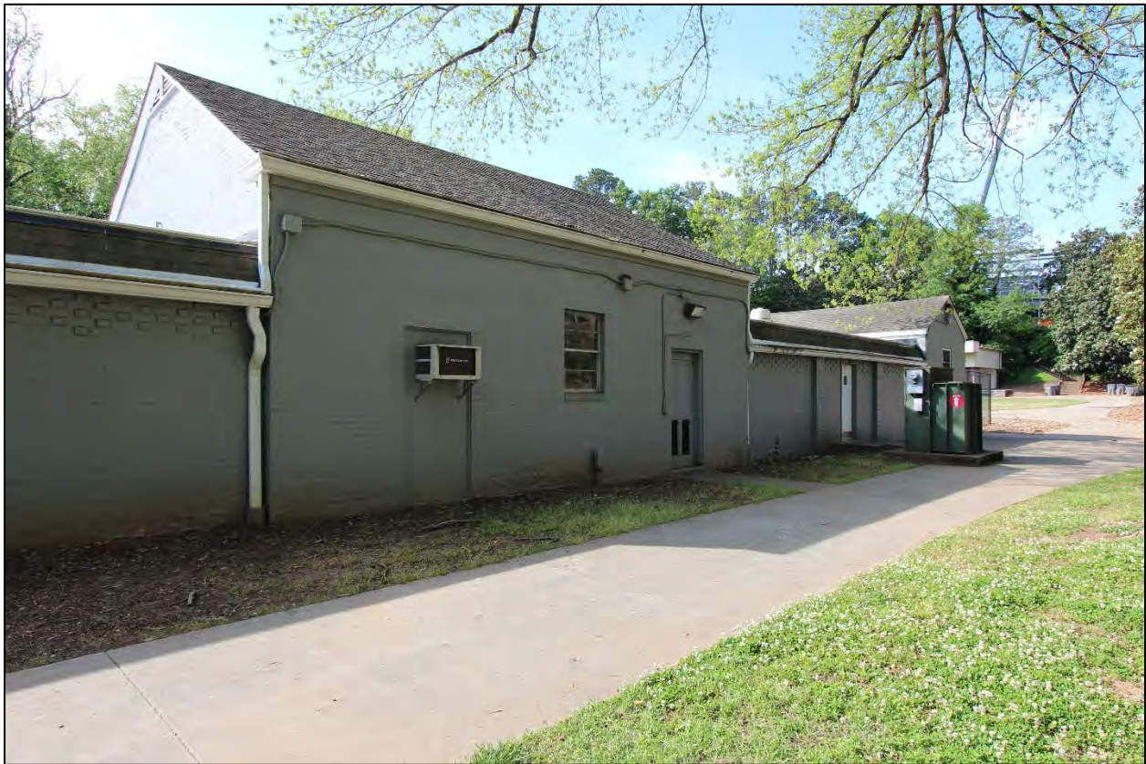
Figure 3.10 Pool House, rear elevation detail, facing south.
