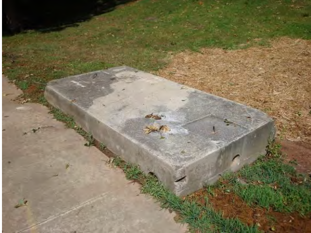
Image 67: Backwash Holding Tank
