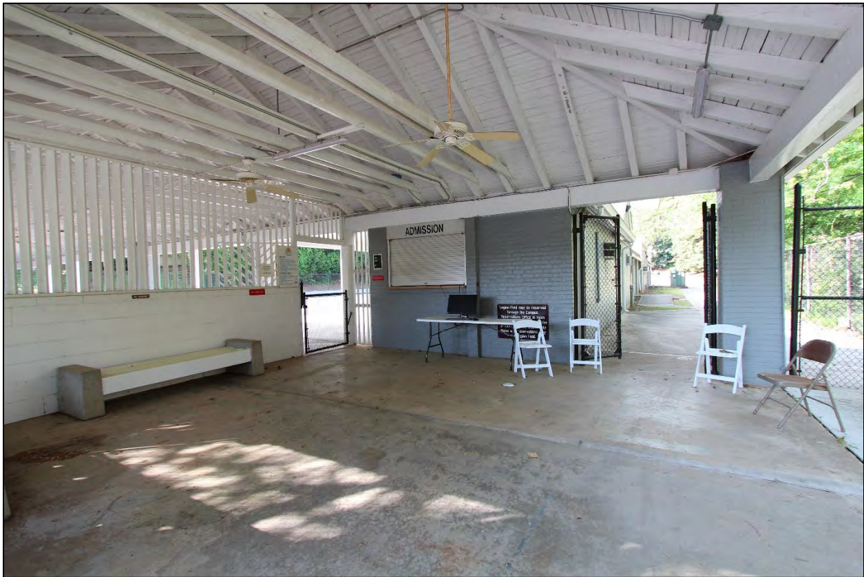
Figure 3.22 Pool House, main entry to pool area, facing southwest.
