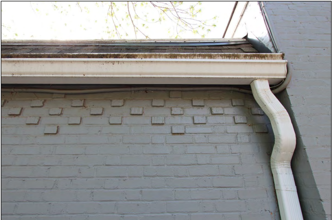
Figure 3.9 Pool House, rear elevation, brick detail, facing southeast.
