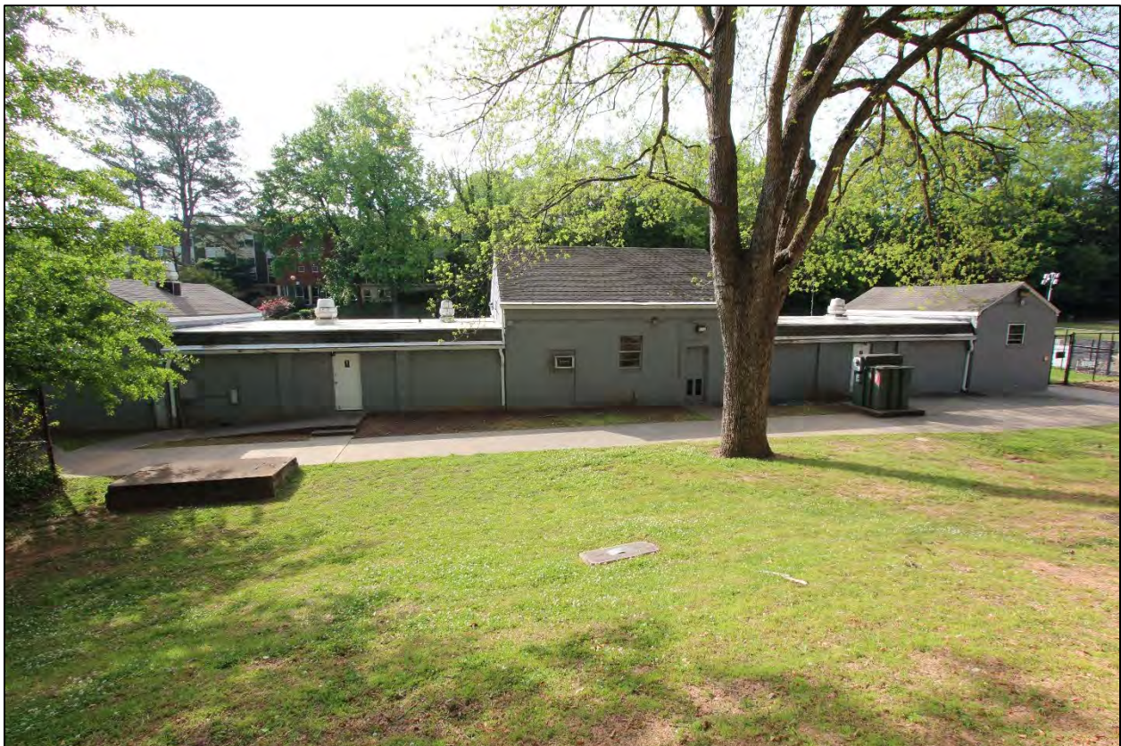
Figure 3.5 Pool House, rear elevation, facing south.
