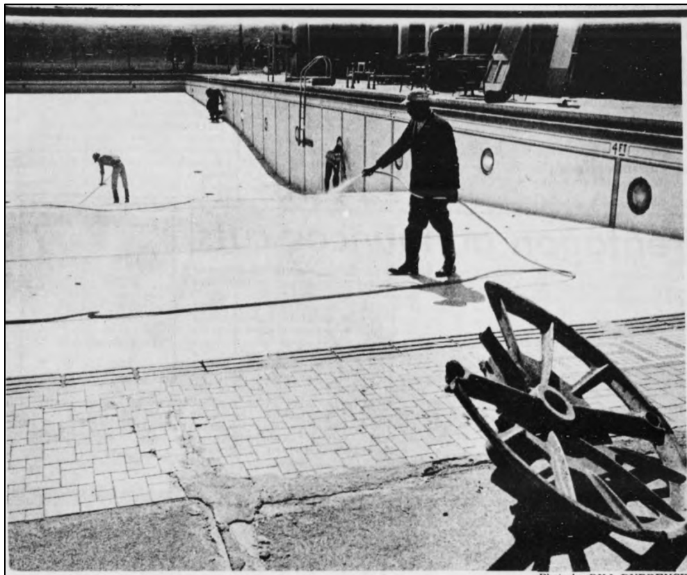
Figure 2.10 Cleaning of Legion Pool, 1973. Note original tile at pool ledge ( Red and Black April 17, 1973).
