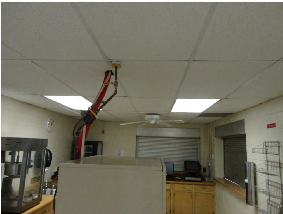
10. Typical mercury-containing fluorescent light bulbs in Concession room.
