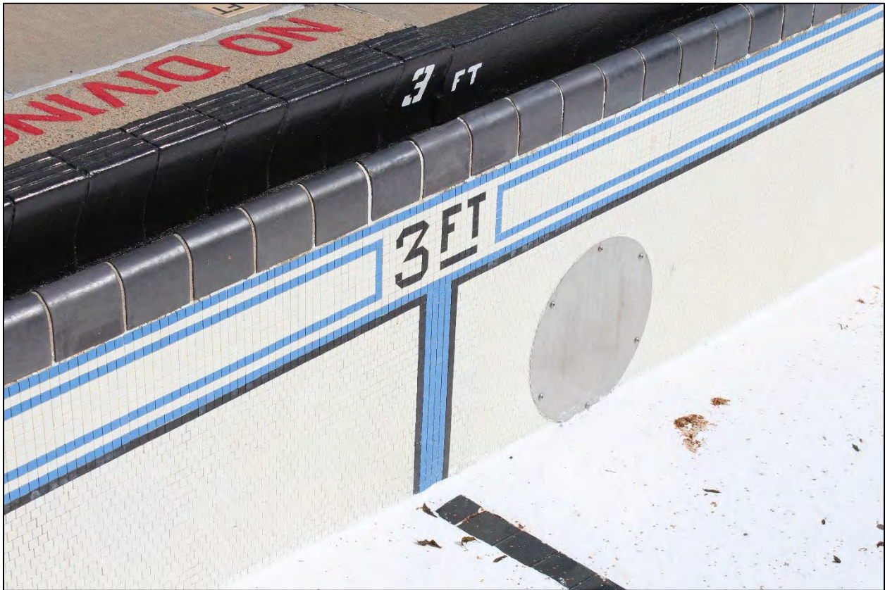
Figure 3.14 Pool tile detail at west end.
