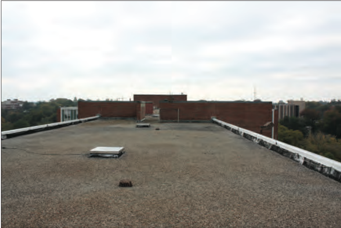
A. North Tower Parapet Wall
