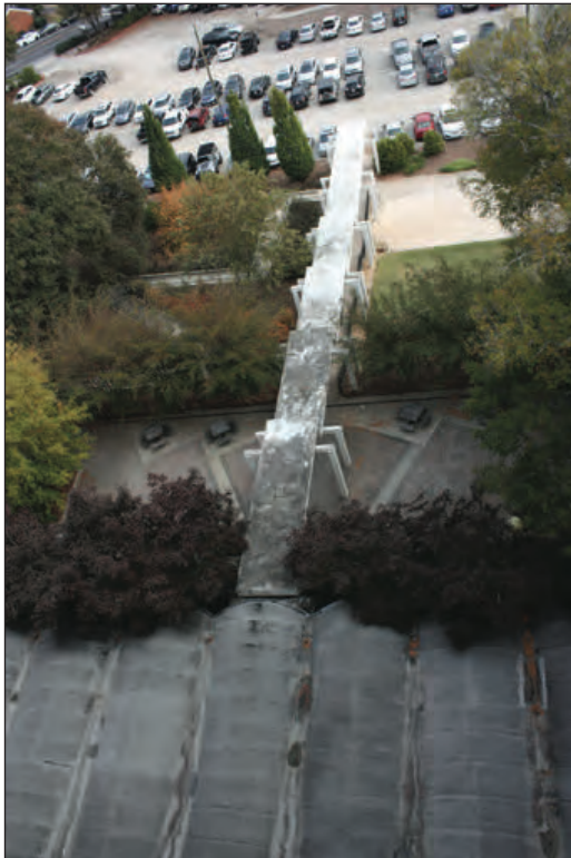
B. Rooftop View of Walkway
