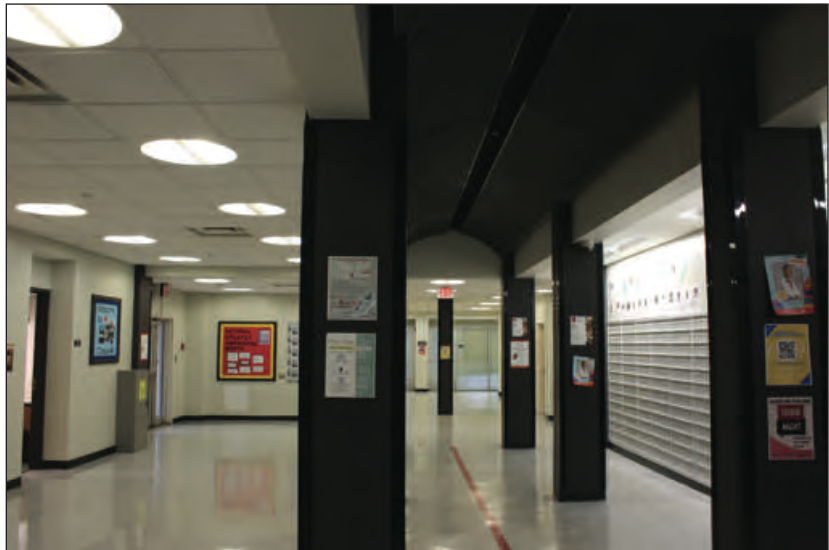
B. Covered Barrel-Roof Ceiling
