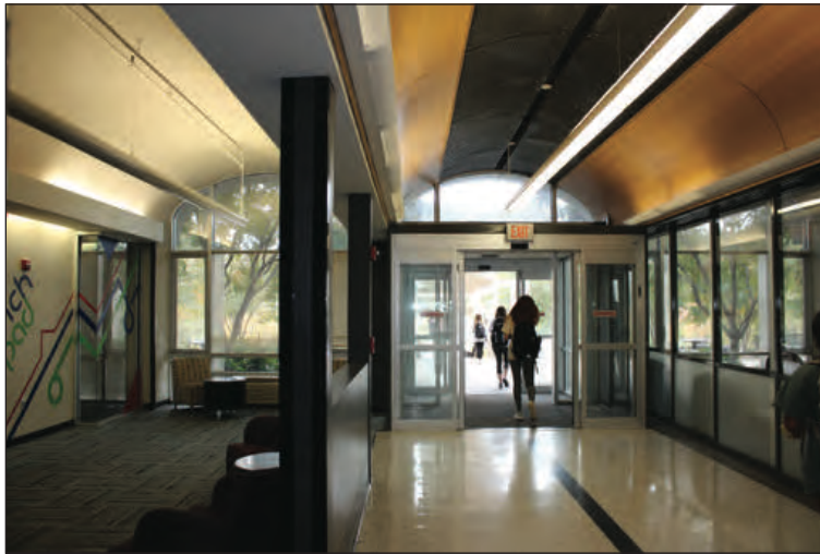
A. Partially Covered Barrel-Roof Ceiling
