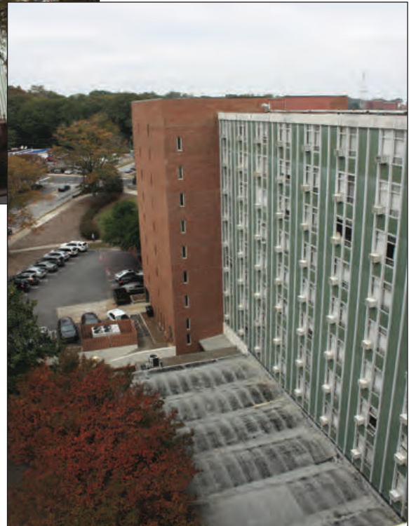
C. North Tower, South End of Southwest Elevation
