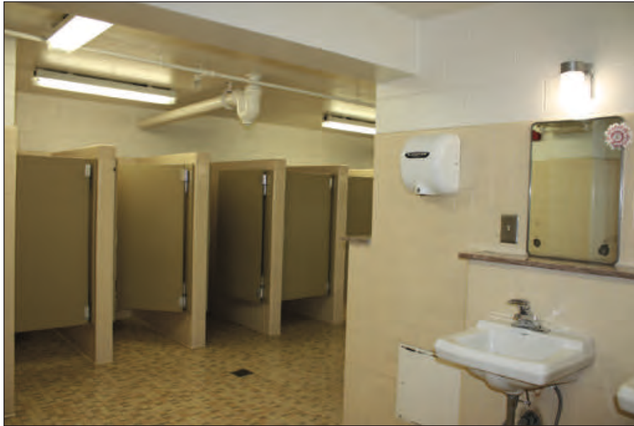
A. Shared Toilet Stalls and Sinks
