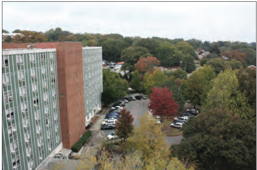
B. Rooftop View of Northeast Elevation Parking Lot
