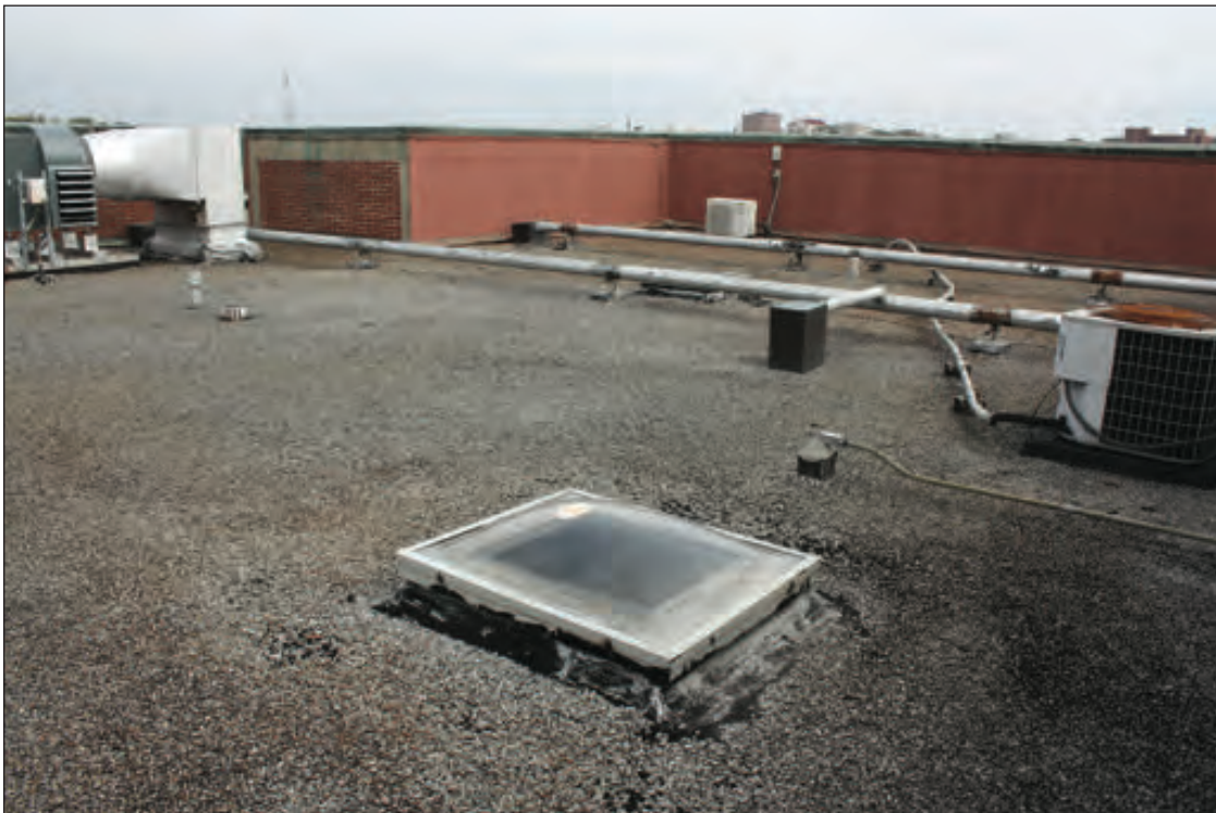
B. South Tower Parapet Wall Interior
