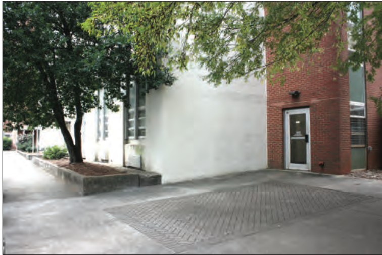
A. North End of North Tower
