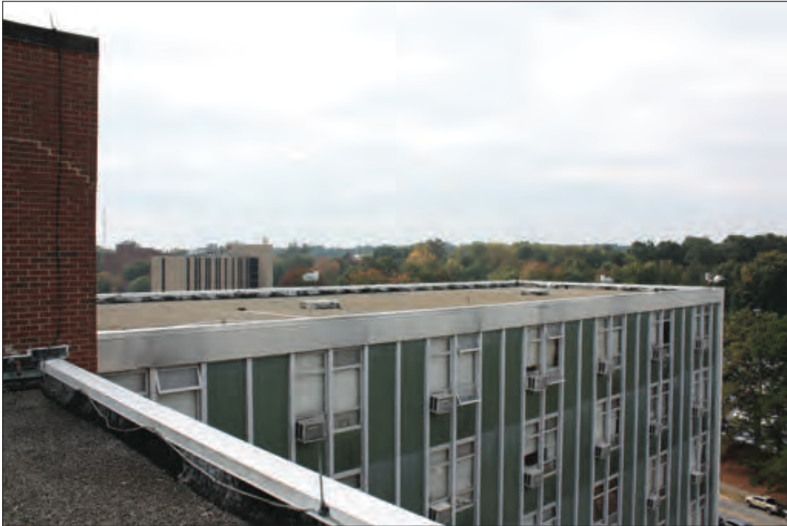
A. View from North Tower Roof toward South Tower Roof
