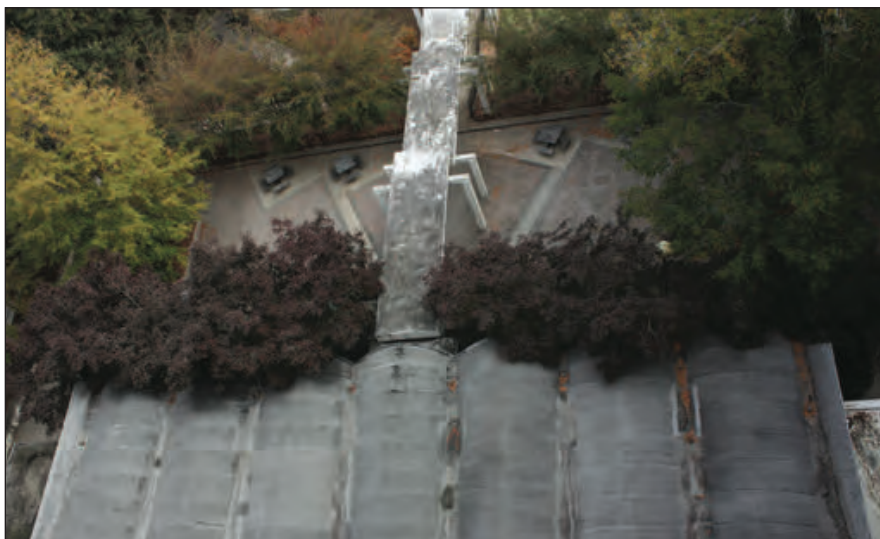
C. Rooftop View of Northeast Elevation Entrance Wing
