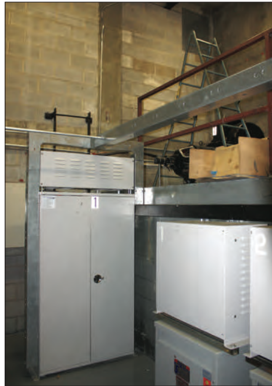
B. General Use Elevator Machines
