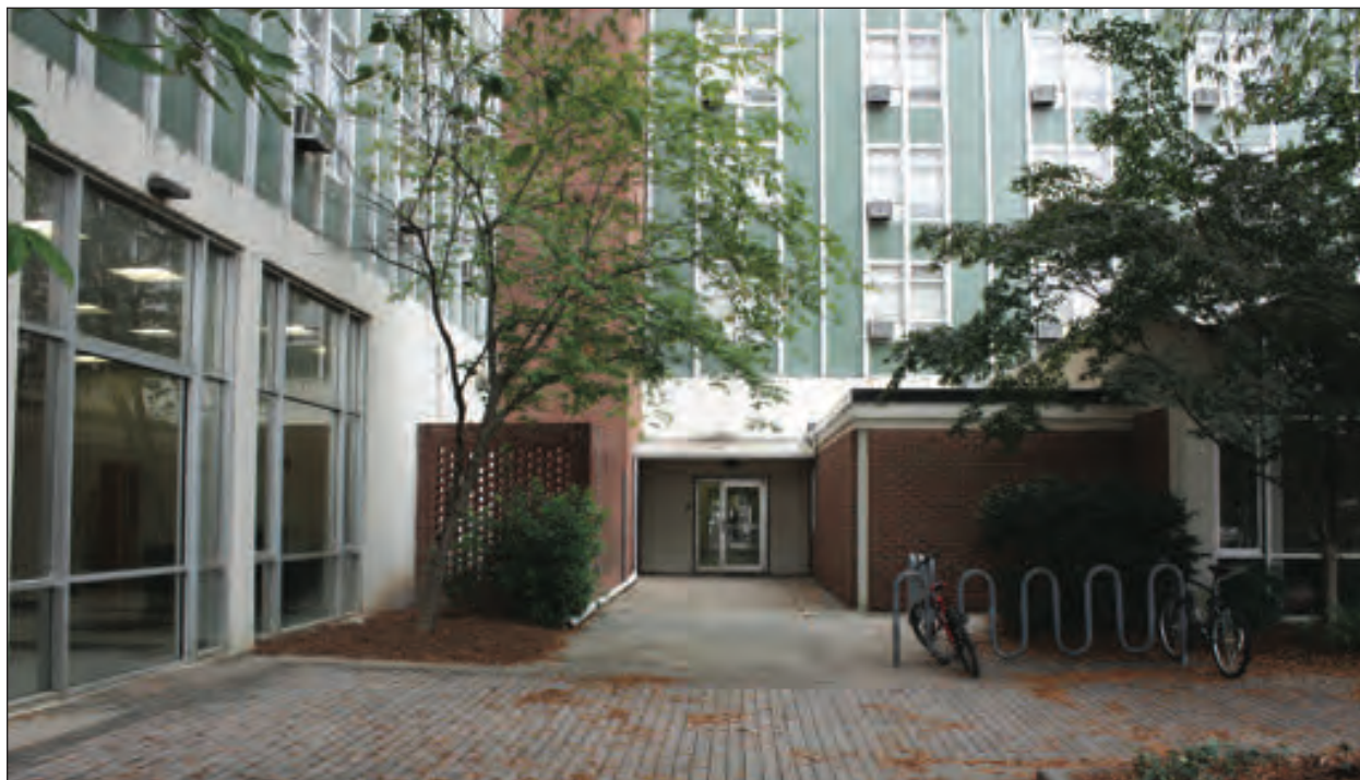
A. Juncture of South Tower and Northeast Elevation
