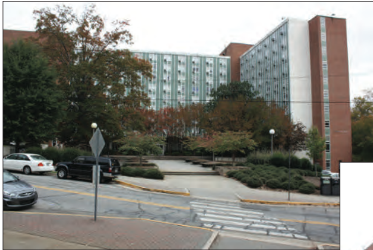
A. Southwest Elevation Approach
