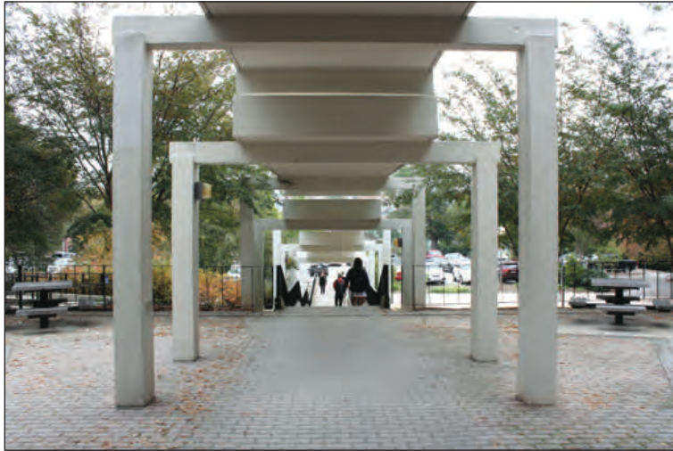
A. Walkway View Below Canopy
