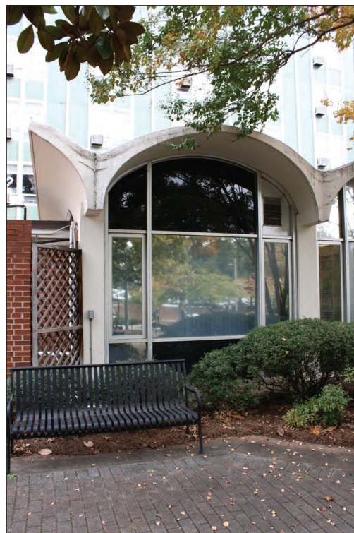
B. Window Bay, Southwest Elevation
