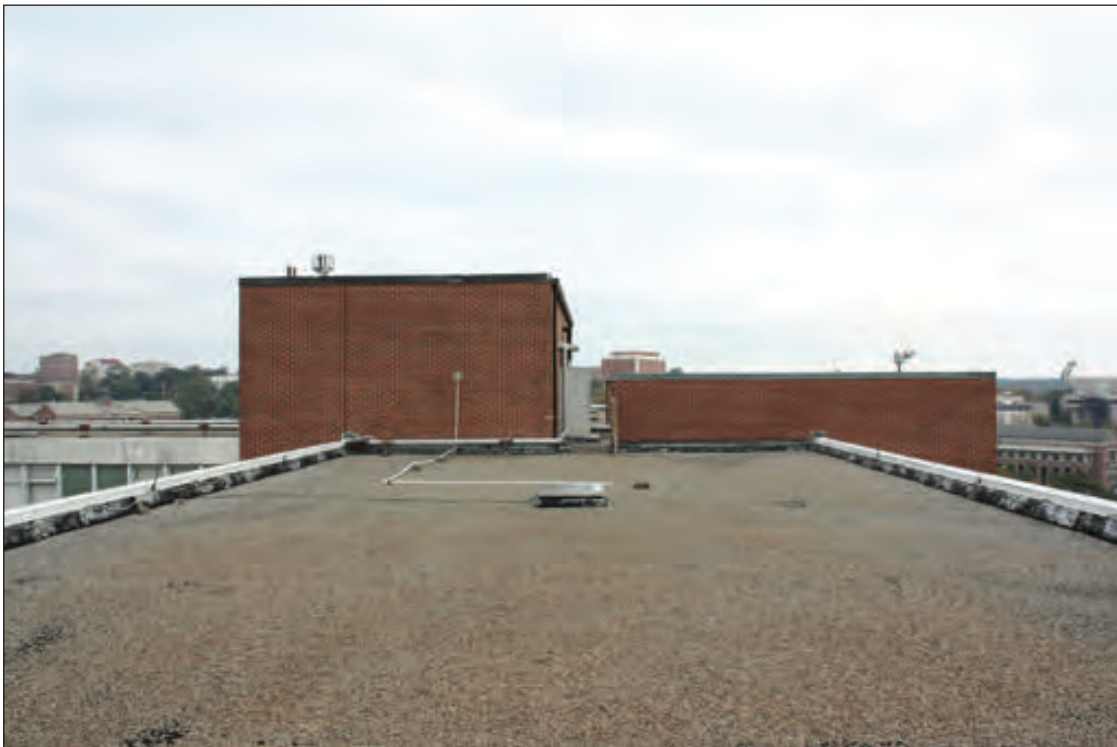
B. South Tower Parapet Wall and Rooftop Equipment Room
