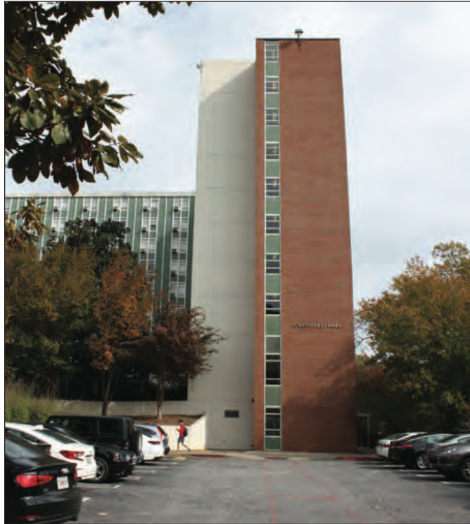
A. Stairwell Panels, Southwest Elevation of South Tower
